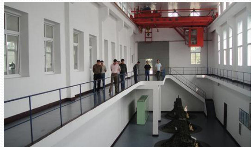
Pump Station Operation
