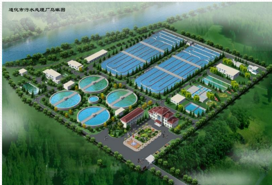
Hebei Zunhua WWTP and wastewater recycling project Design treatment capacity of 80000m 3 /d
