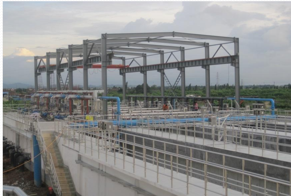
Jiangmen Jianghai WWTP Design treatment capacity of 80000m 3 /d
